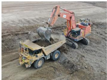
Figure 1: Bulk Earthworks – 180 tonne excavator loading Cat 777 Rigid Dump Truck
